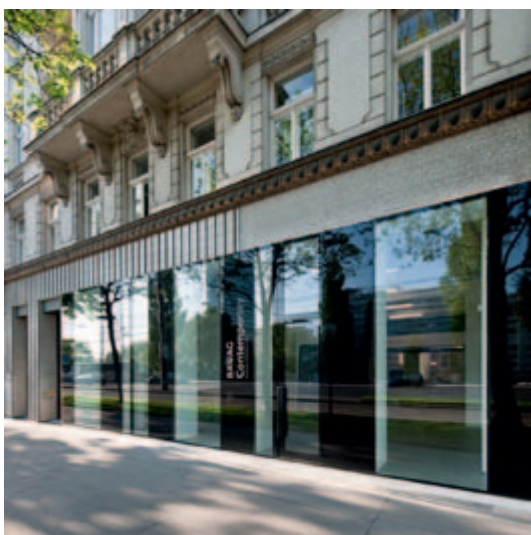
Exterior view of the BAWAG Contemporary art space
